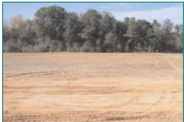
New Football/Soccer Field Under Construction
